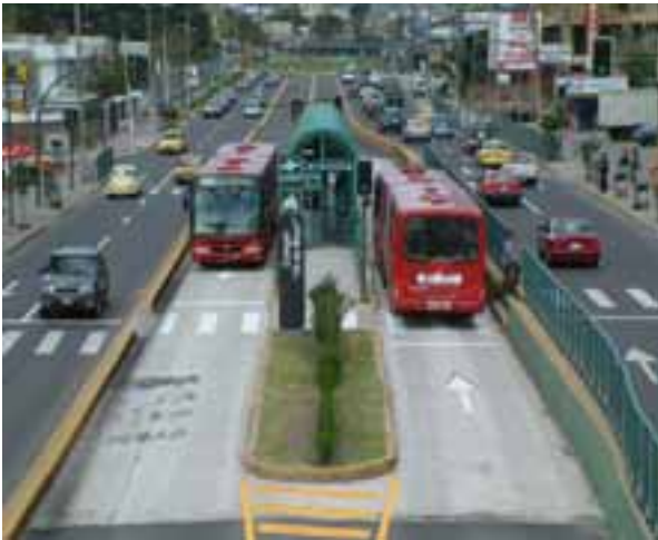
Figure 3.4: Median busways and station in Bogota
